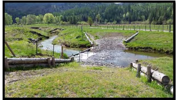
The 400 lineal feet of stream bank reconstruction completed in 2014, connected to the 800 feet completed in 2013, and the 400 feet completed in 2012; totals 1,600 lineal feet of stream bank restoration.
